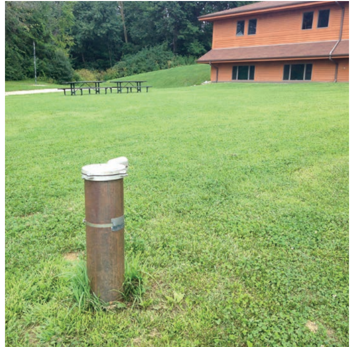
Properly located and constructed wells prevent contaminants from moving down into the drinking water source
